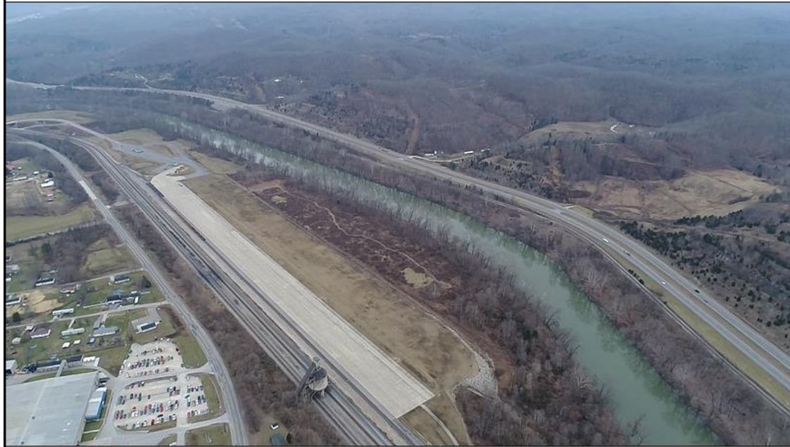
Figure 2 Aerial View of the HIG Facility
